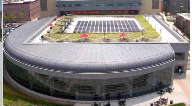
Photovoltaic System on Roof of NJIT
