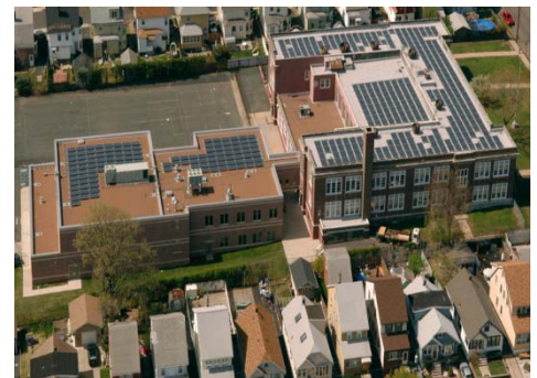
137KW Photovoltaic Array at Schuyler School
