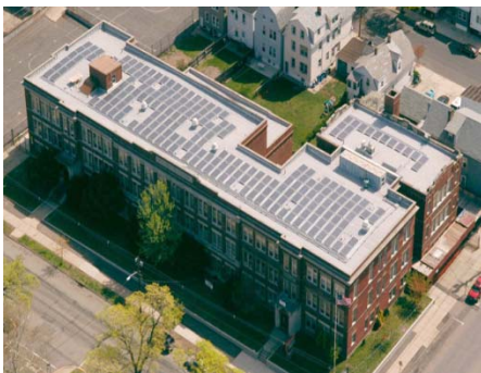
89 KW Photovoltaic Array at Garfield School
