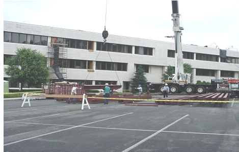
Exterior of Building
